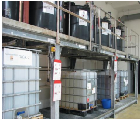
Figure 1: Storage class compatibility check used in Germany (source: Technical Rules for Hazardous Substances TRGS 510)
